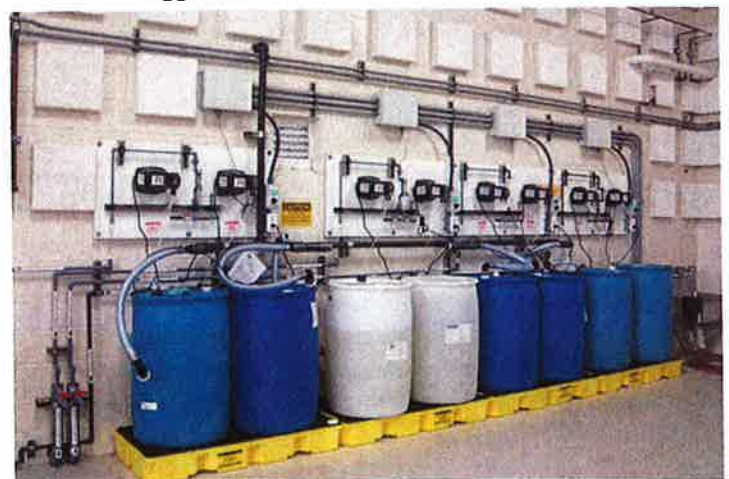
Sodium hydroxide is added in order to raise the pH of the treated water, sodium hypochlorite (bleach) is added for disinfection, and a trace amount of ammonia is added to form a longer acting disinfectant in the distribution system.
